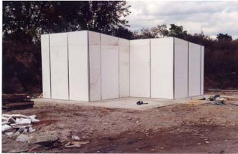
2. Lightweight aluminum channels also are used at the corners and between every 4-foot by 8-foot panel to hold them in position during spraying. From start to finish, all of the foam panels for the walls and roof can be installed and ready to be covered by Grancrete cement in just a few hours.
