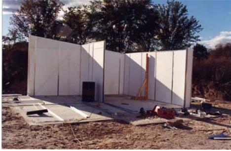
1. The shell of the building is constructed using expandable polystyrene (EPS) foam panels, such as Styrofoam-brand EPS panels, which are held in place using lightweight aluminum channels anchored to the foundation.
