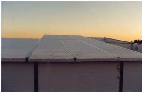
3. The roof is also constructed of foam panels that are held in place by aluminum channels. Once covered with Grancrete, the roof becomes an integral, water-tight part of the home.
