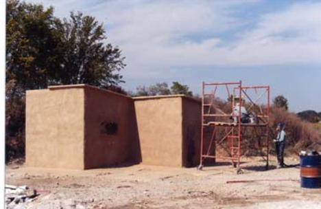
5. Both the exterior and interior of the walls and roof are sprayed to a thickness of about one-half inch. Grancrete is sprayed around the windows and door frames to ensure a weather-proof seal.
